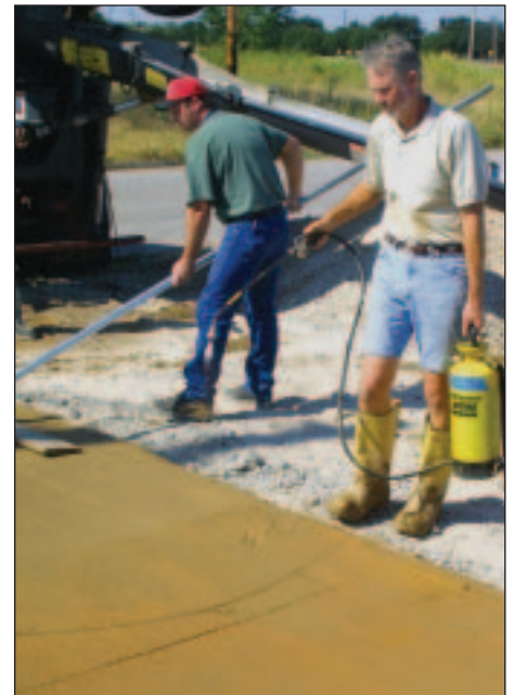
Doug Bannister applies Control Finish, the newest aid in controlling the set.
